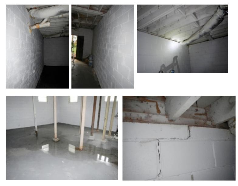
Front wall bowed due to soil and moisture loads. Wall under-designed. Require reduce moisture at center front outside wall
